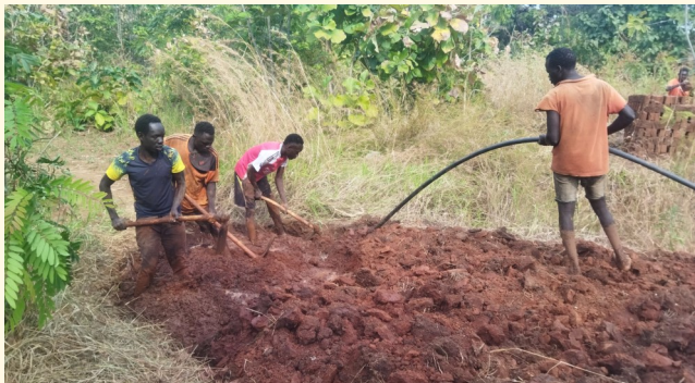
Busi Joseph (Green & Yellow T-shirt) with his team mixing mud for laying bricks
